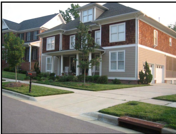
Wood Shingles and Clapboard Siding
