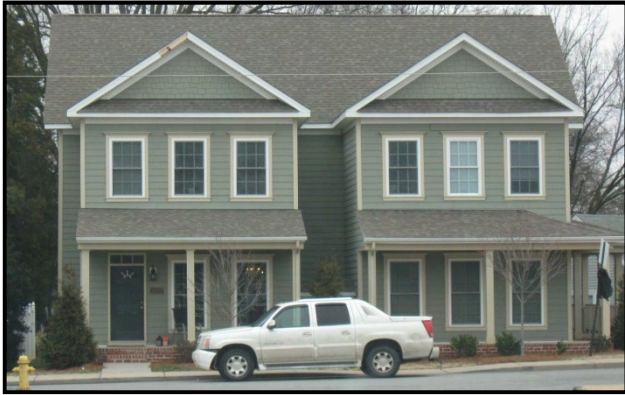
Entrances on Different Plane of Façade
