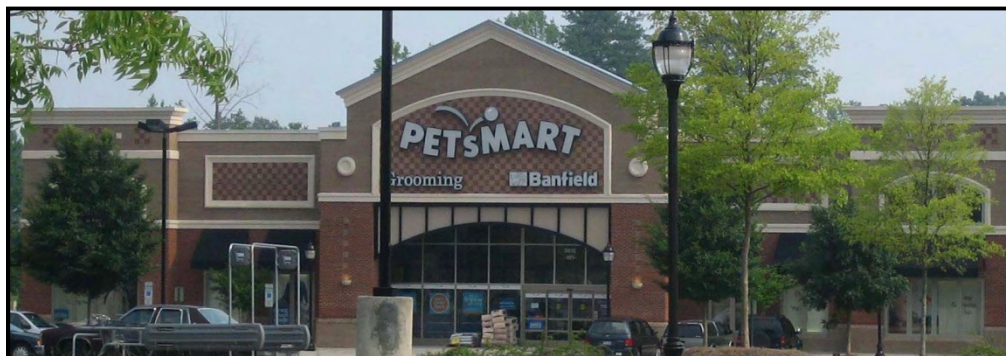
Facade with Recesses & Projections
