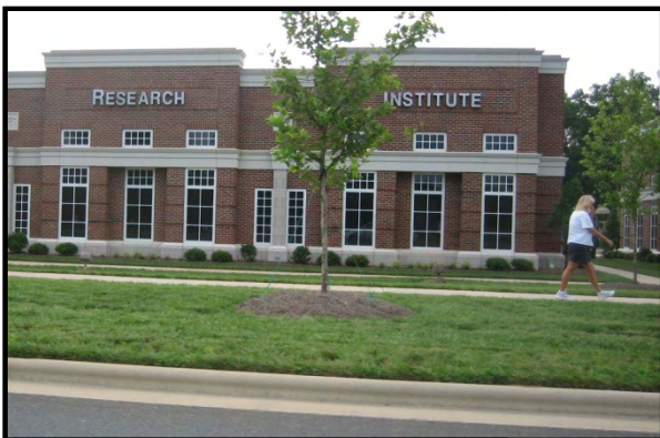
Parapet with Decorative Cap & Varied Roof Line
