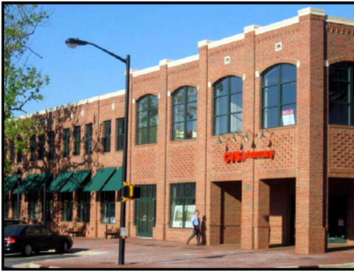
First Floor Windows
