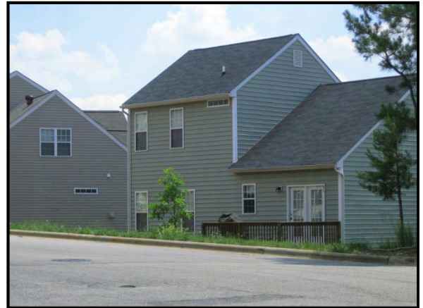
Less than 9-inch Overhang
